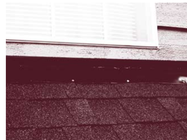
New roof-to-wall flashings.
